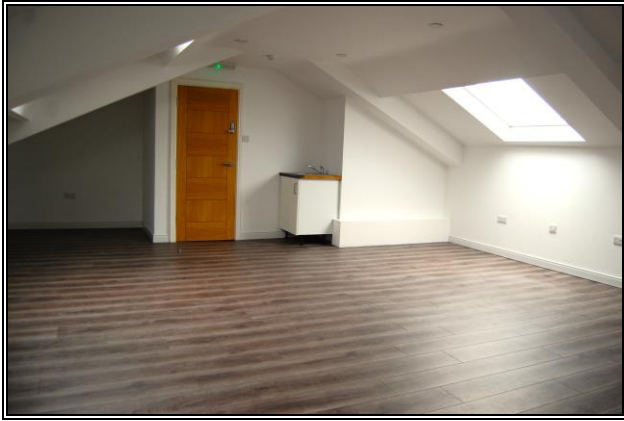
Second Floor Office 2
